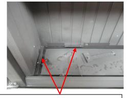
Ensure that the left hand log is sitting on top of the 2 support brackets (NOT directly on Burner)
