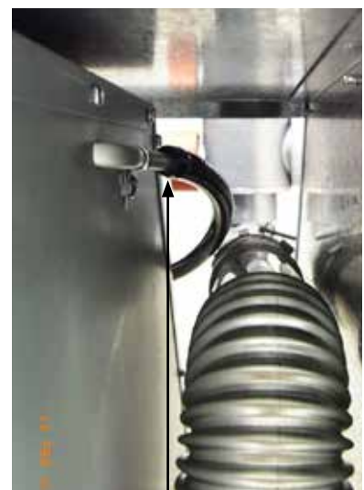
Flue condensate pipe connection
