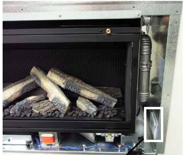
Commissioning sheet—located inside a plastic pouch inside the unit (right hand side)
