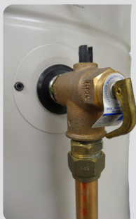
TPR position - top of cylinder
