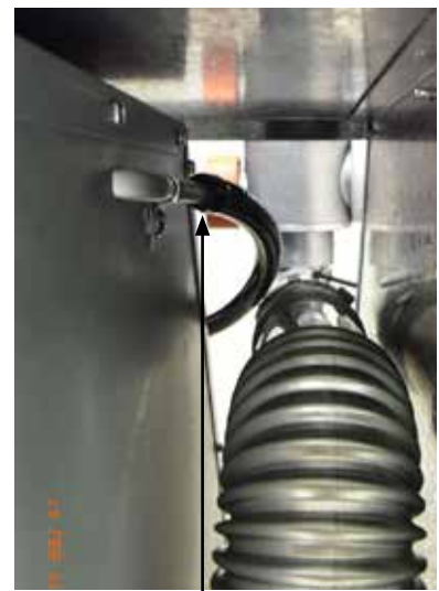
Flue condensate pipe connection
