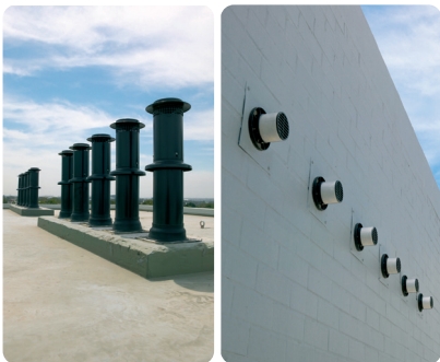
Older style roof cowl and horizontal terminals all terminating at the same height
