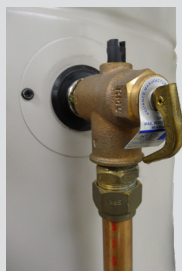
TPR position - top of cylinder
