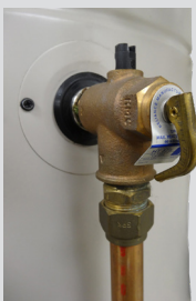
TPR position - top of cylinder
