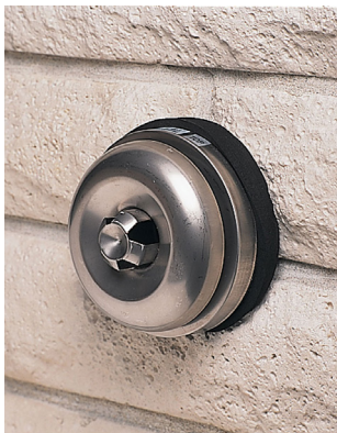
Mushroom flue terminal on a brick wall
