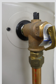
TPR position - top of cylinder
