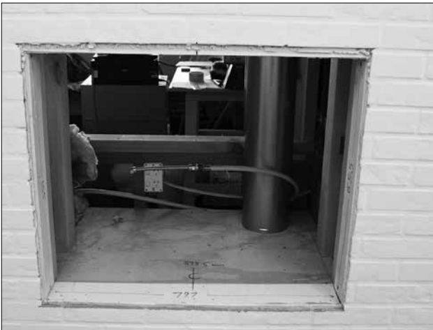
Mock chimney enclosure
