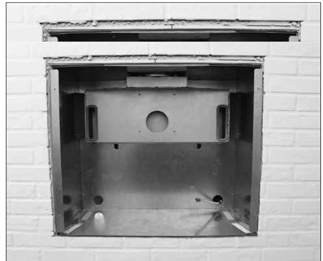
Zero clearance box and coaxial flue adapter
