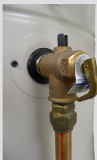
TPR position - top of cylinder
