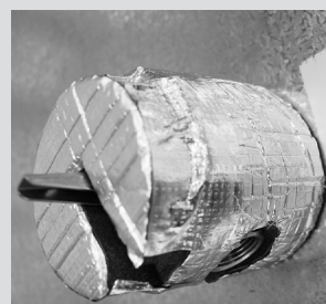
Insulated TPR valve for the 250 and 300 L cylinders
