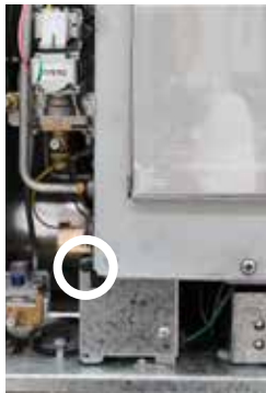
Black screw in lower bracket
