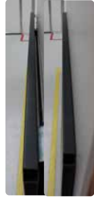
Outer frame mounted on tabs
