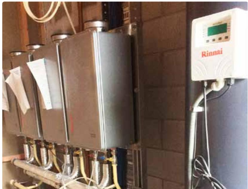
*The system offers the flexibility of sizing the appropriate number of Rinnai INFINITY water heaters and different hot water storage capacities to supply specific hot water volumes.*
