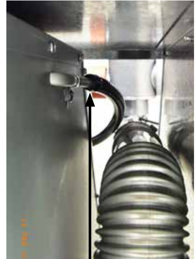
Flue condensate pipe connection
