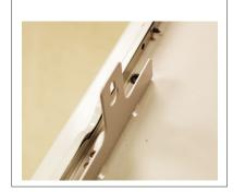
**8.** A-Series, slide water heater under back pocket in the recess box, and align with keyhole on the top mounting bracket.
