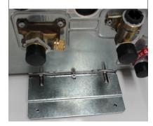
**6.** Secure the HD56kWe lower mounting bracket.
