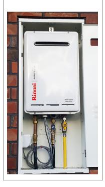
**Final**: Recess box installed and sealed.
