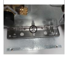
**5.** Slide the HD56kWe lower mounting bracket in place.
