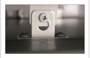
**4.** Secure water heater bracket to lower adapter as pictured.
