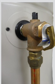
TPR position - top of cylinder
