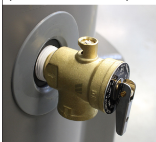
TPR near top of cylinder (insulation not fitted)
