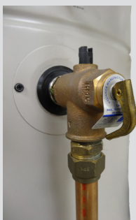
TPR position - top of cylinder
