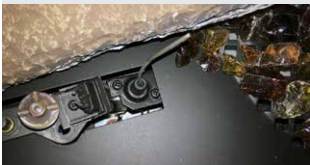
Flame rod CLEAR of metal log fibres.
