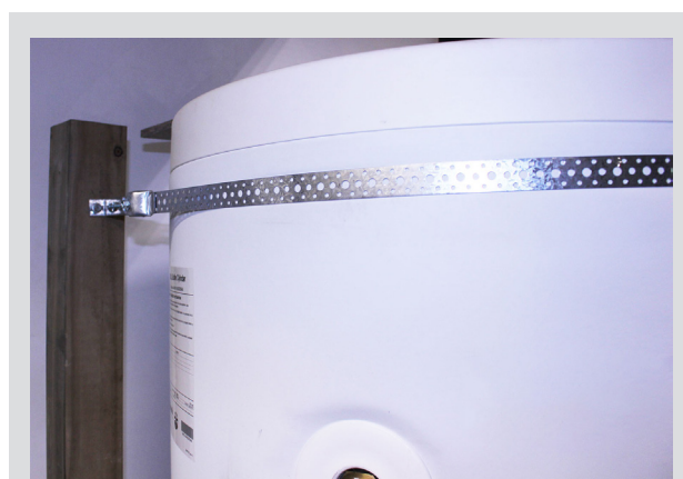
Seismic restraint needs to be determined by a calculation specific to the installation, as per NZS 4219.
