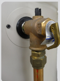
TPR position - top of cylinder
