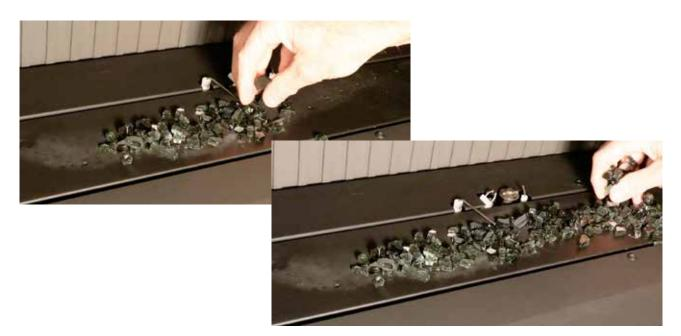
Start the fire and make sure that the flames track across the entire burner bed. Move the glass around as required.
