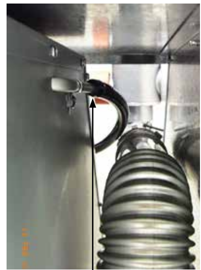
Flue condensate pipe connection
