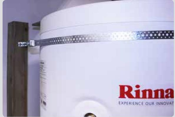
Seismic restraint needs to be determined by a calculation specific to the installation, as per NZS 4219:2009.
