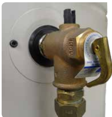
TPR position - top of cylinder
