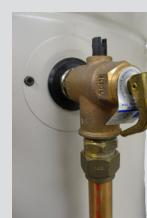
How to operate the easing gear
