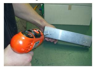
2. Install the diverter on the flue terminal ensuring it clips into the top and bottom lip of the terminal.
