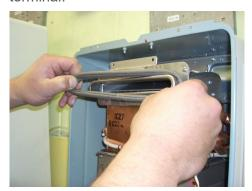
3. Remove the inside three screws from the flue terminal and set aside.
