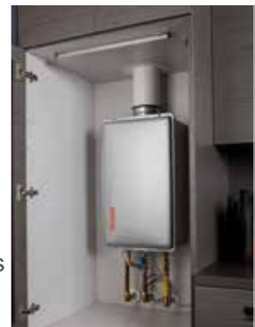
Example of an internal unit installed in a cupboard - Rinnai Auckland showroom
