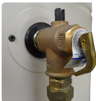
TPR position - top of cylinder
