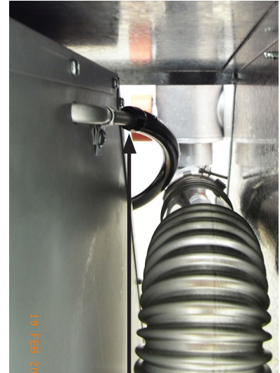
Flue condensate pipe connection
