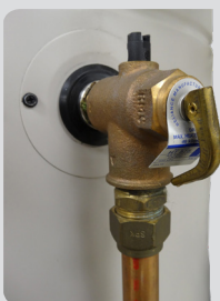
TPR position - top of cylinder
