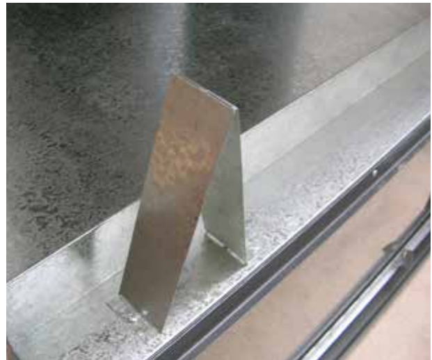
Step 2: Bend and secure the metal standoffs
